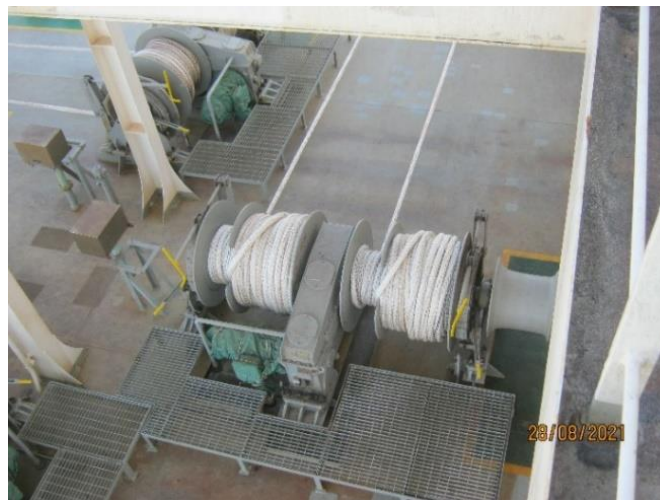
Fig 14: Multiple layers on a split mooring drum
