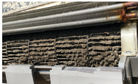
Presence of mould, fungus and mildew in the air conditioning systems
