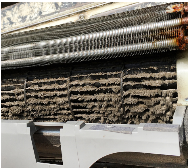
Growth of mould, fungus and mildew in the air conditioning systems
