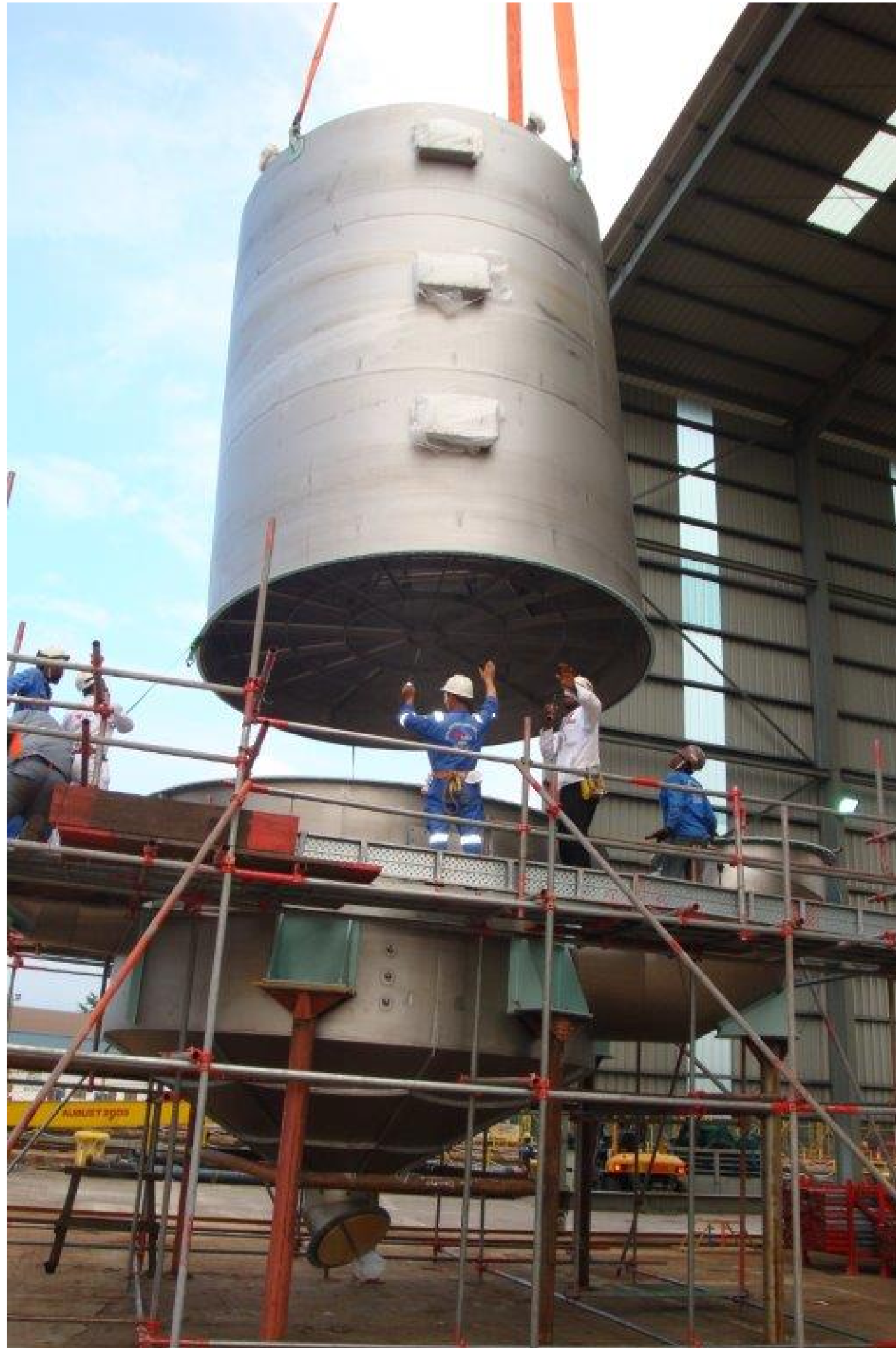
Picture on left : Scrubber installed on the new funnel
