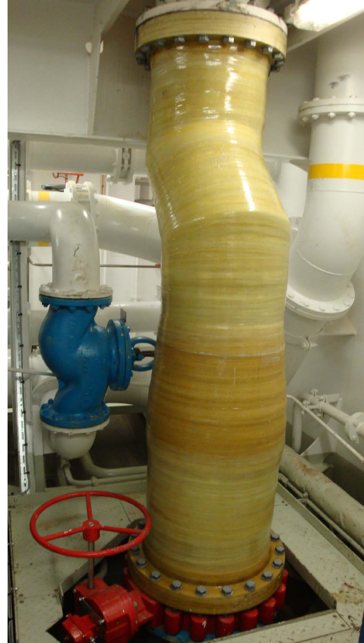
Picture on right : GRE Piping – A critical part in scrubber installation
